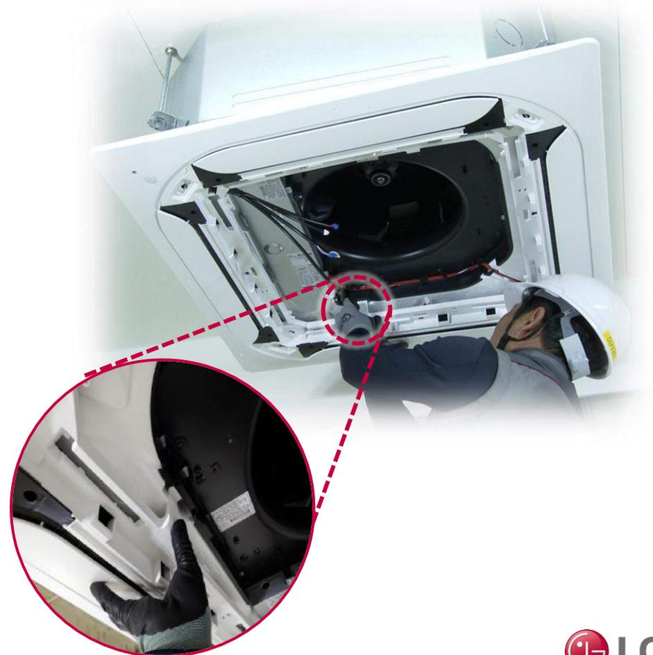
Drain Leakage Check
